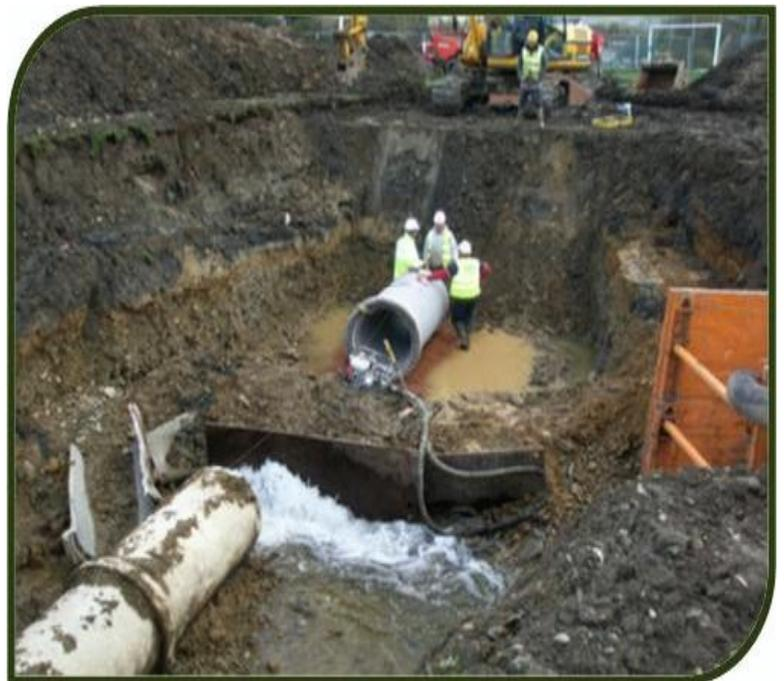
**SUB-STANDARD CULVERT BEING REPLACED**
