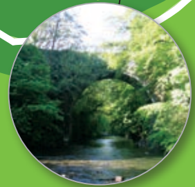
The Penllwyn Tram Road Bridge Pont Dramffordd Penllwyn
