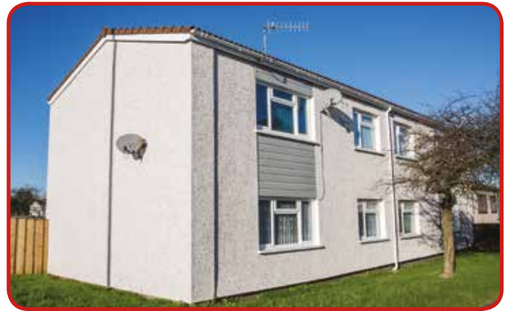
Lansbury Park homes after energy efficiency works.
