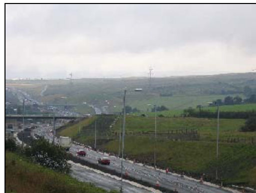
Photo 2 – View of SW of site from opposite side of A465
