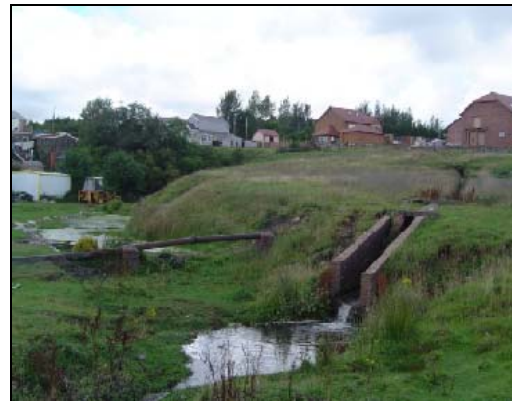
Photo 6 – Main watercourse running through site
