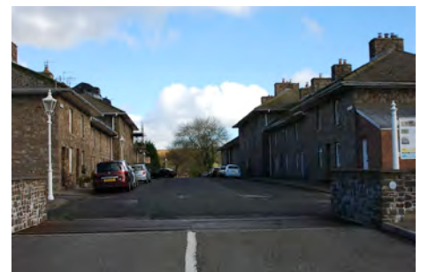
The well-proportioned wide street between Middle and Lower Rows is a strong feature of the area, but the large expanse of macadam is without warmth or texture.
