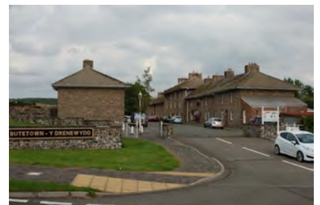
Entrance to Bute Town off the A469 with large sign, stone walling and cattle grid
