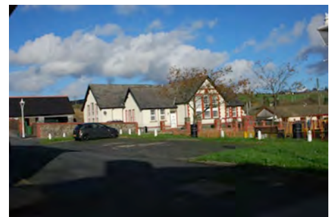
View of the old school facing the playground
