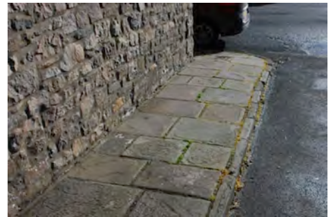
Pennant flagstone paving recently reinstated is entirely appropriate and adds to the character of the area.
