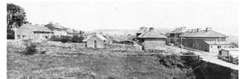
View of Bute Town prior to 1970's refurbishment works with bridge over railway
