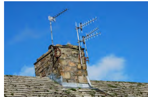
Chimney stack on Middle Row with a plethora of television aerials
