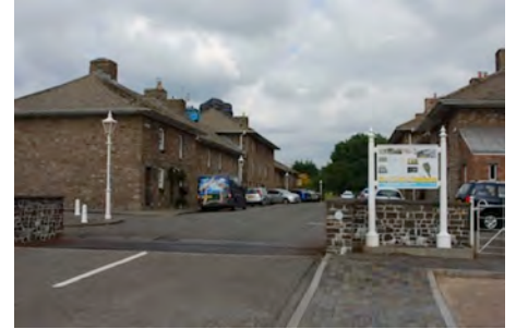
View of street between Middle and Lower Rows, where haphazard parking and vehicles mar the view of the street, even during the working day when many residents are not at home.
