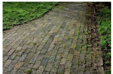
Pennant stone setts have been used in recent works and work well with the overall aesthetic of Bute Town
