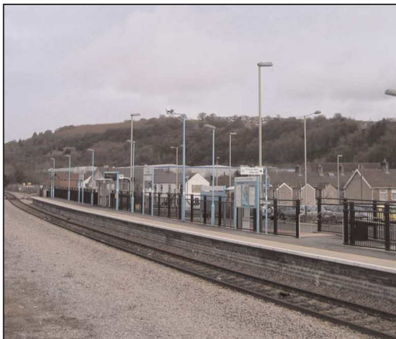
Newbridge Station Platform
